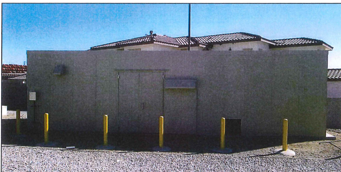
Completed installation of sound enclosure (facing south)
