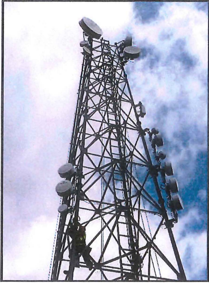
6B Tower – New Receiving Dishes
